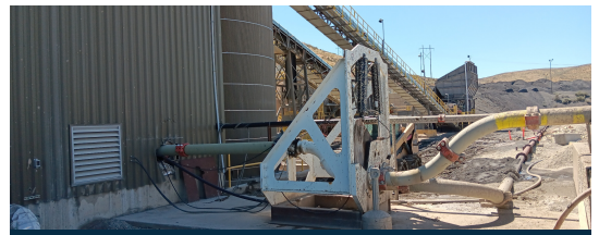
ON-SITE TECHNICAL SUPPORT
